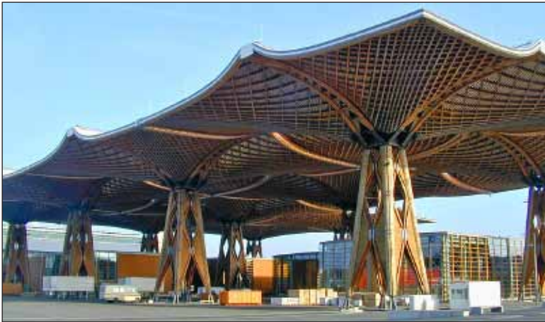
Free-standing wooden roof built for World Expo 2000, Hannover, Germany. Credit: Wikimedia.
