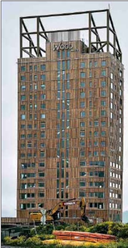
Mjøstårnet building, Brumunddal, Norway (during construction) with 18 storeys for mixed use. Credit: Wikimedia, Oyvind Homstad.
