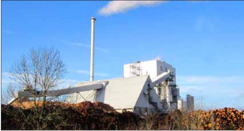
Electricity generator fueled with waste wood, on site of a sawmill.
