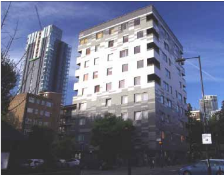
Stadthaus : a nine storey wooden apartment block in London. Upper left is a concrete and steel apartment tower; lower left is an old brick built apartment block of low cost accommodation.
