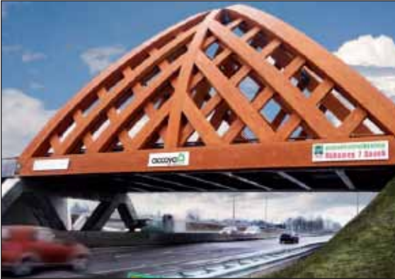
Wooden bridge over an autoroute in the Netherlands constructed with 'Accoya' treated glulam beams. Credit: Wikimedia.
